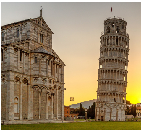
Leaning Tower of Pisa
